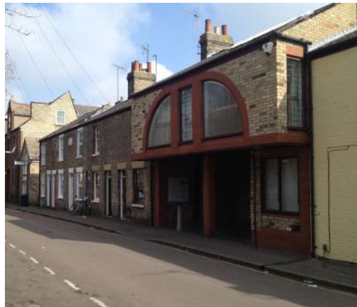
'Before' views Views of internal alley and street (Photos: Rowan Haysom)
